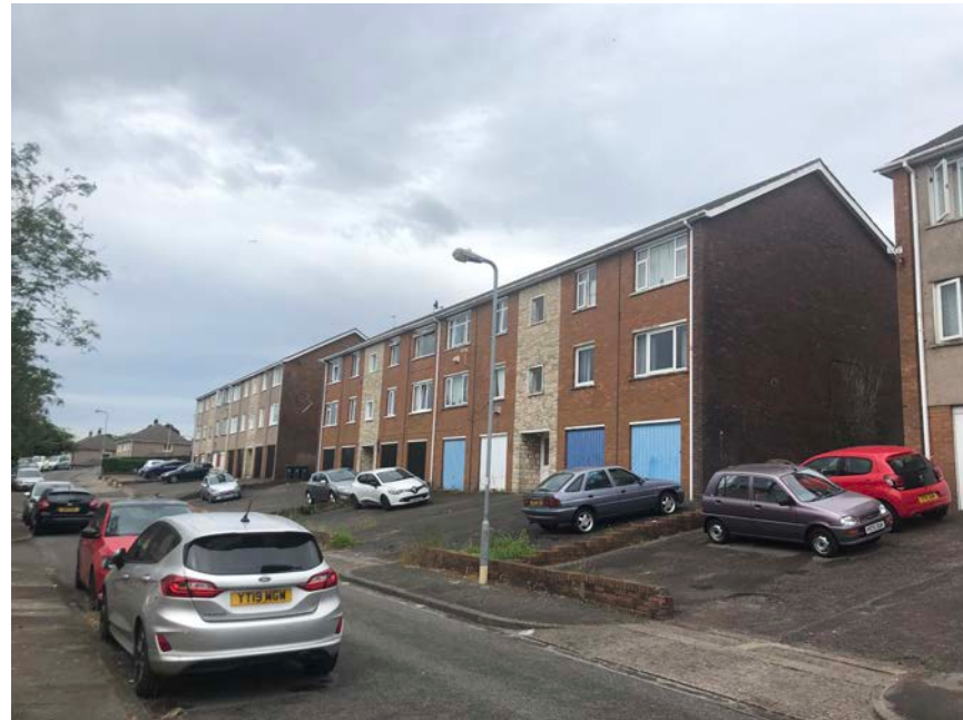
(A) Buildings A, B & C viewed from Lynmouth Crescent facing North East
