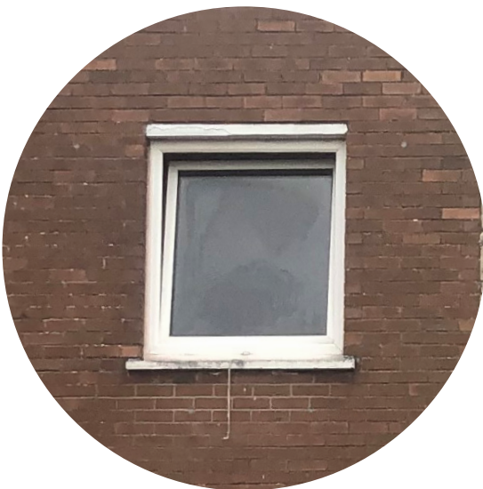
UPVC framed double glazing
