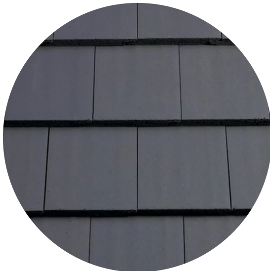
Hung tiles to suit existing
