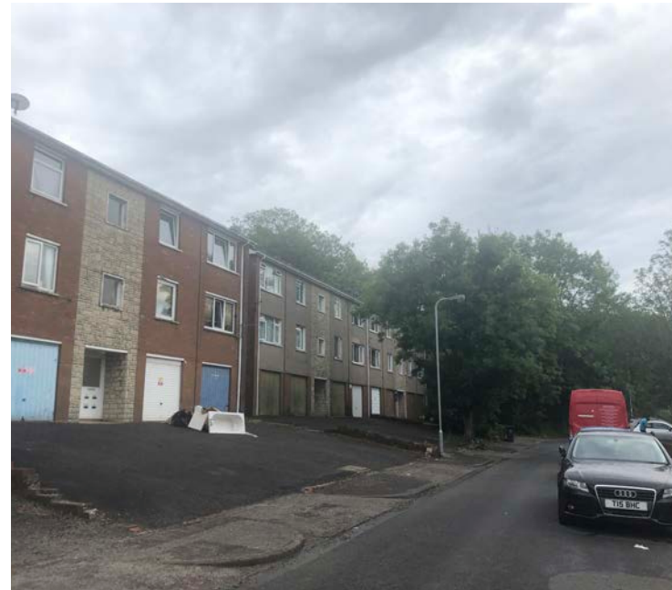
(B) Buildings D & E viewed from Lynmouth Crescent facing South East
