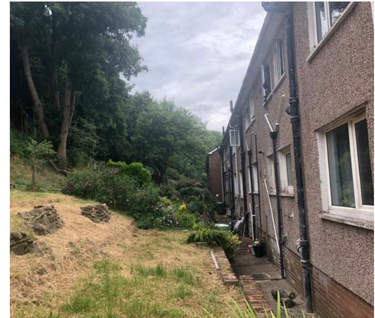
(C) Rear sloping gardens behind buildings A to E.
